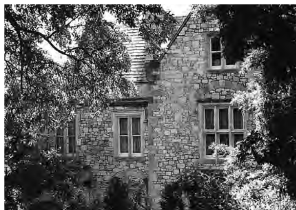
Larkbeare House, Topsham Road
