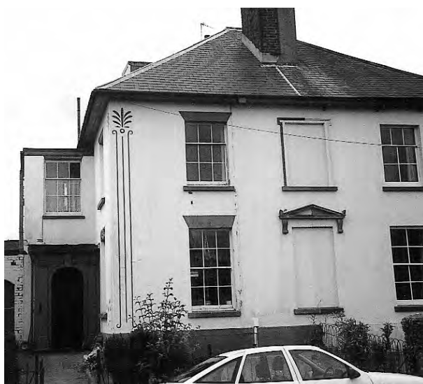
Listed house in Friars' Walk
