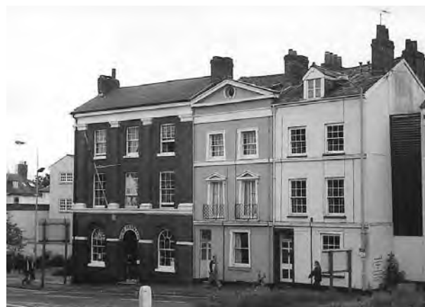
Nos. 71-73 Holloway Street
