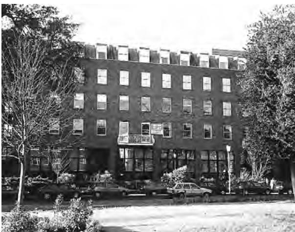
Broadwalk House, Southernhay West
