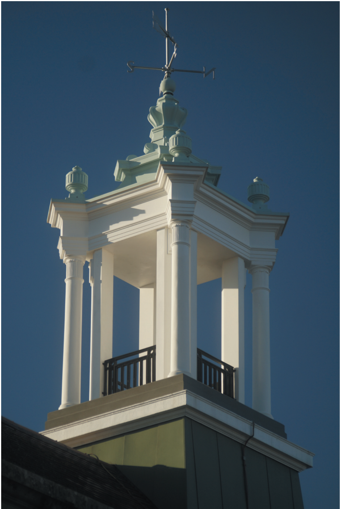
The rear elevation of Central Station, Exeter, with the replacement cupola in position.
