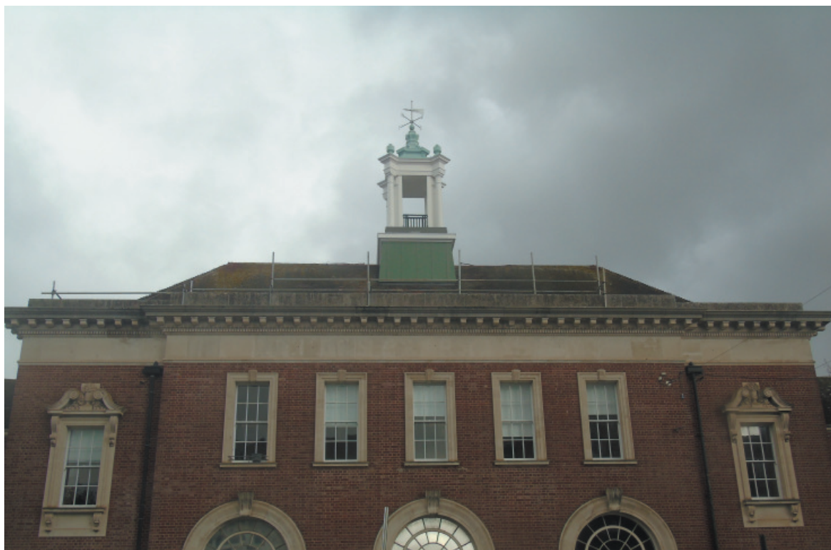
The front elevation of Central Station, Exeter, with the replacement cupola in position.
