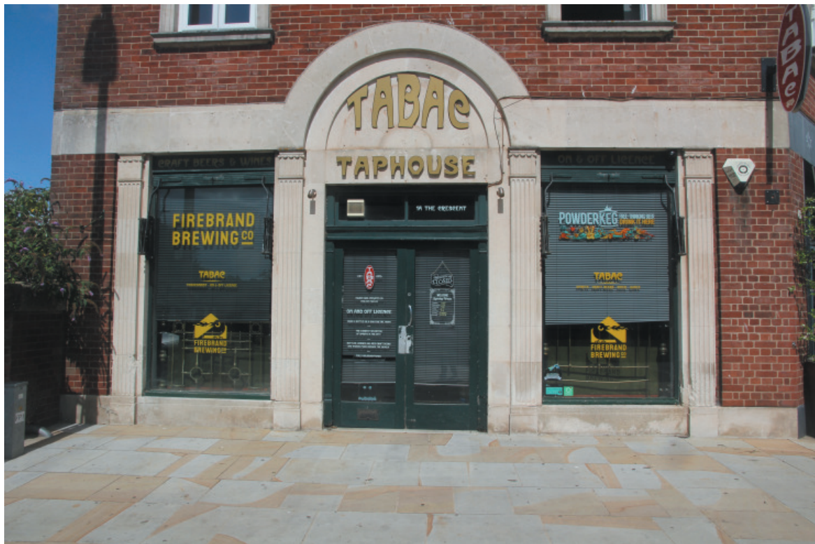
Fig.13. The shop front into the north end pavilion.
