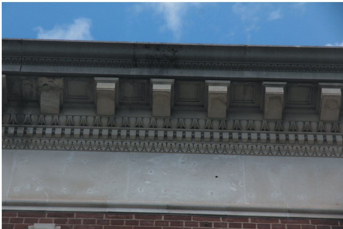
Fig.10. Freestone details: the entablature with a dentil cornice and orders of moulding.
